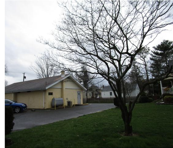
The parking spaces along the south side of the building can be converted into pervious pavement to allow stormwater runoff from the roof and pavement to infiltrate the ground. Downspout planter boxes can be installed on the north side of the building to capture runoff from the roof and enhance the aesthetic of the building. A preliminary soil assessment suggests that more soil testing would be required before determining the soil's suitability for green infrastructure.
